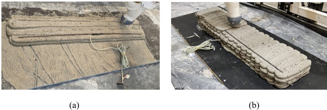
Figure 12. (a) Printing of the 3D beam with longitudinal (b) and transversal printing direction, with insertion of the instrumented bar.
