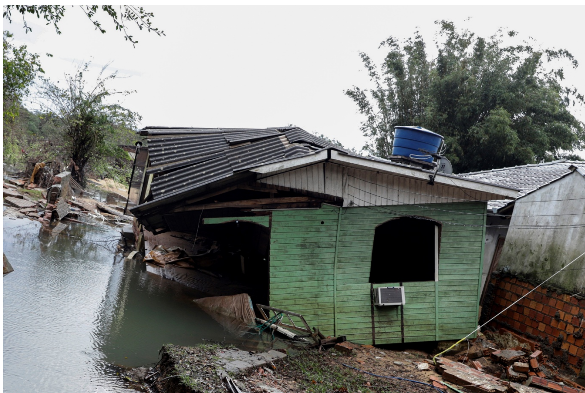
Figure 1 Houses destroyed on Ilha da Picada after rains and new flooding in Porto Alegre (RS), June 19, 2024 Source: Bruno Peres/Agência Brasil ( https://agenciabrasil.ebc.com.br/foto/2024-06/enchentes-no-rio-grande-do-sul-1718828937 ).
