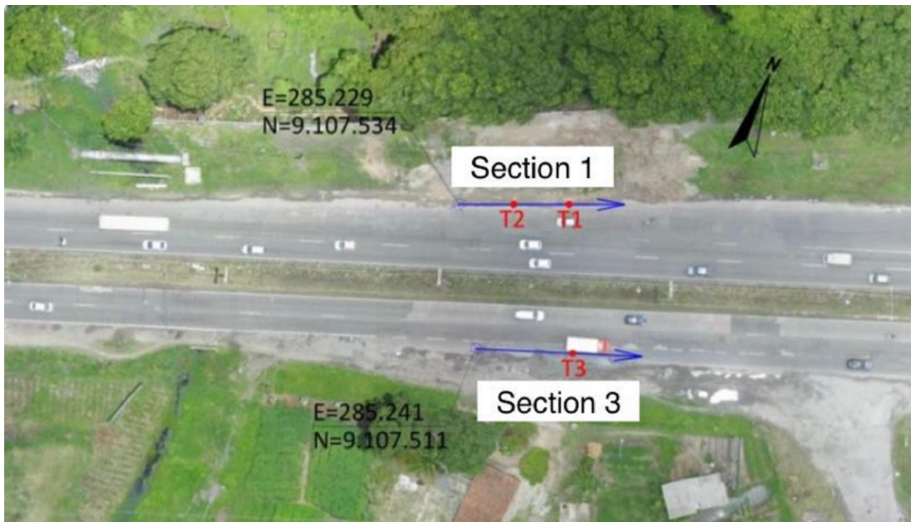
Figure 5: Sections 01 and 03 of the GPR survey
